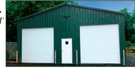
This is a steel-frame building with vertical metal siding. The enclosed area is 30' by 30' and 12' high, plus a covered carport 10' by 30'. This triples the work space for the grounds crew as well as secure storage space for equipment. We now have a good place to work on repairing and refinishing bronze markers, a new in-house service.
